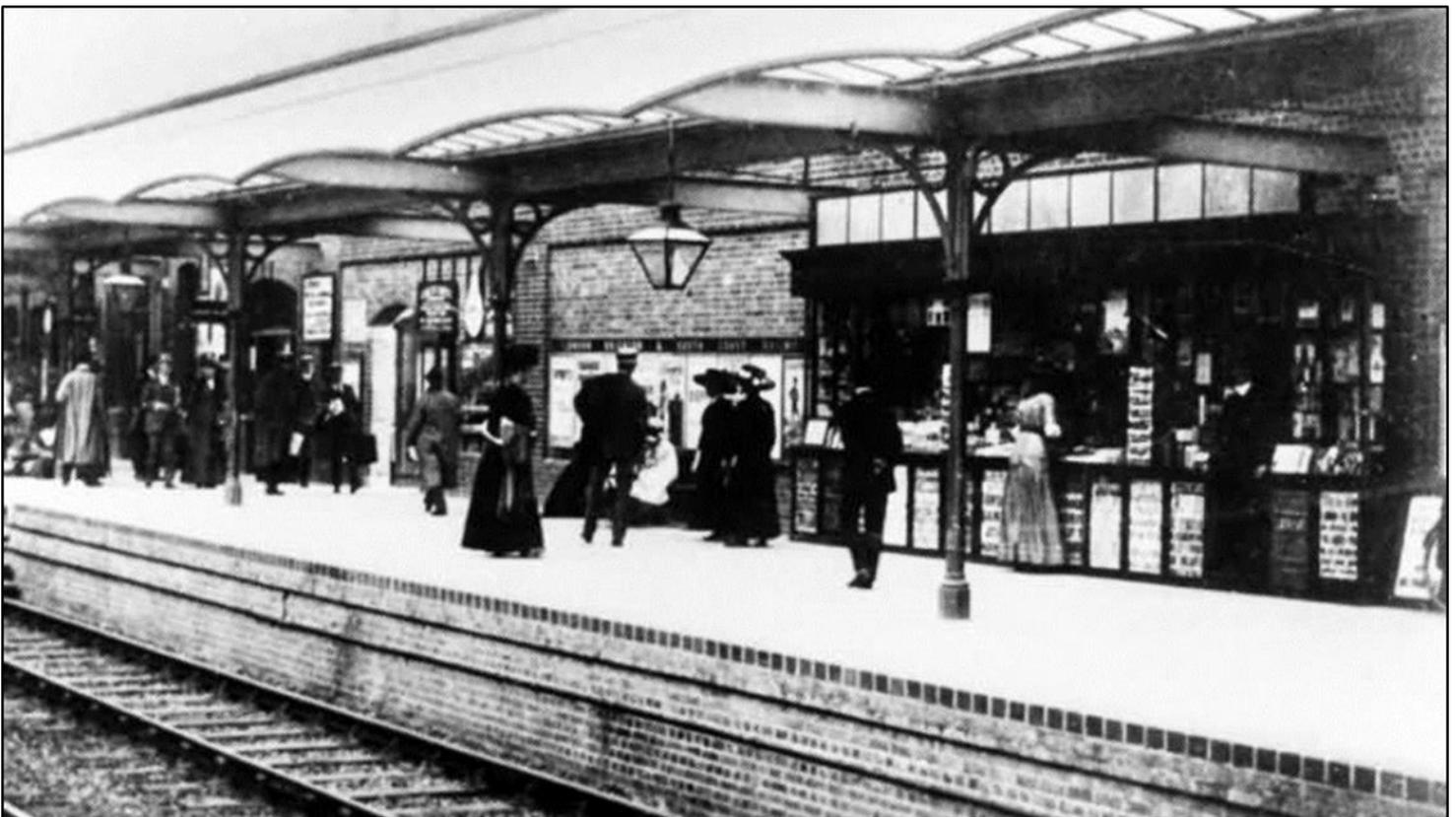
As the line became busier with goods and passenger traffic the infrastructure was improved. The railway was made double track in 1894 and the station, pictured above, was substantially rebuilt and improved in 1905-1907.
