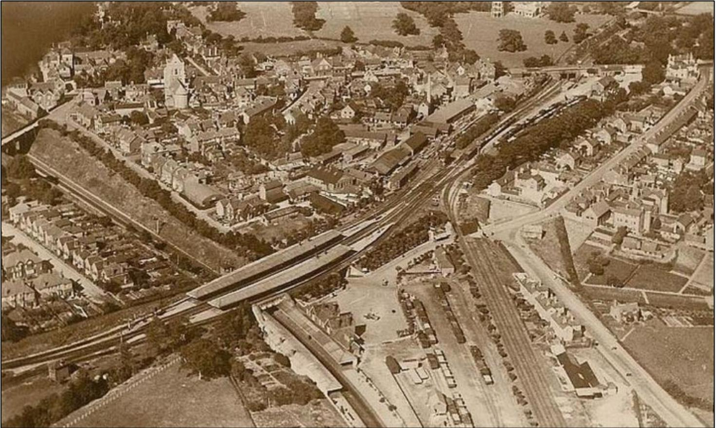
(Above) An aerial photograph of East Grinstead station taken around 1925 showing the two-level station. The railway running across the picture from left to right is the Three Bridges to Tunbridge Wells line, with its high level platforms.
